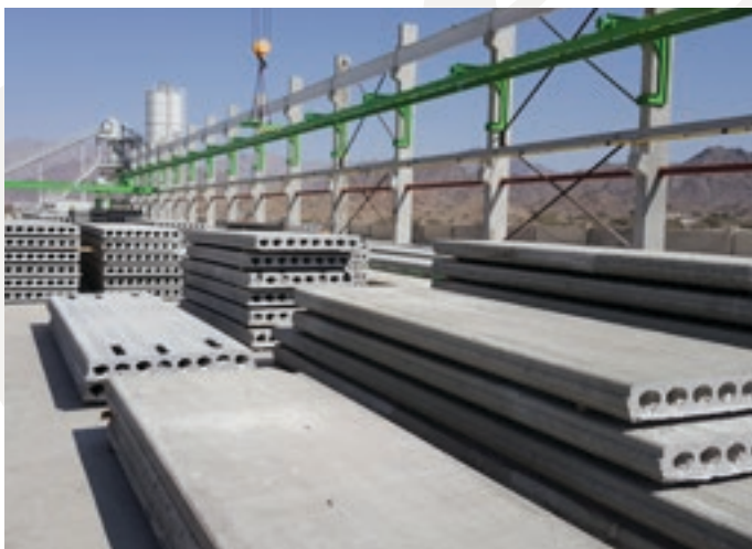
Long-line prestressing beds
